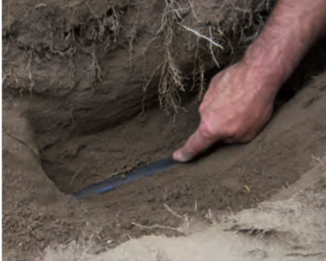
A soil pit has been dug to show the Netafim sub surface drip irrigation system. The dripline laterals are spaced every 1.5 metres.
